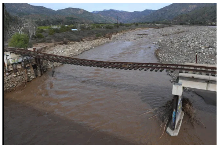
The rail bridge over Sespe Creek just west of Fillmore was damaged by the Jan. 10 storm flows. (photo: County Star)
