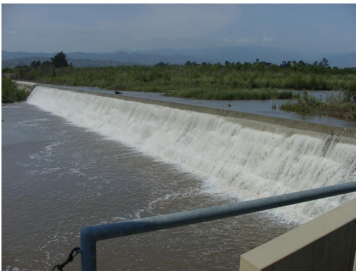
The Vern Freeman Diversion spills 23.5 feet in high flows. The old fish ladder is immediately downstream.
