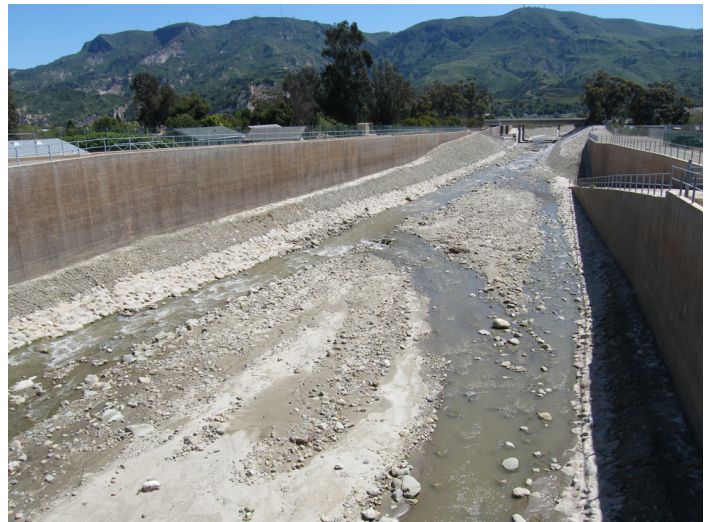
A downstream view of lower Santa Paula Creek, looking towards the freeway bridge. Note how the channel gets narrower as it gets closer to the Santa Clara River. Any wonder why it is flood prone?
