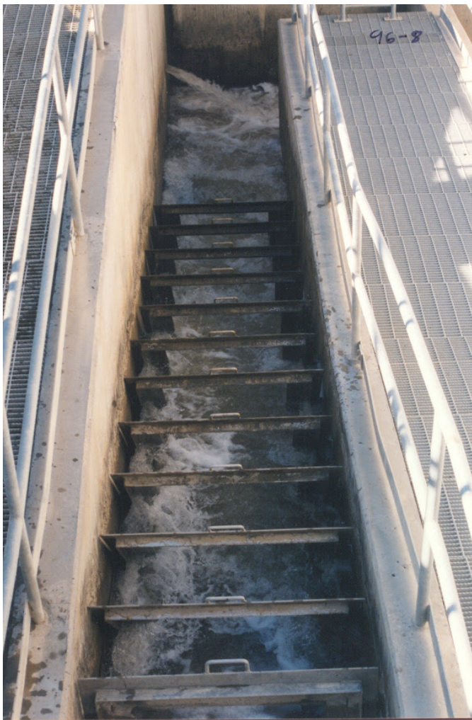
The non-functional fishladder at the Freeman Diversion
